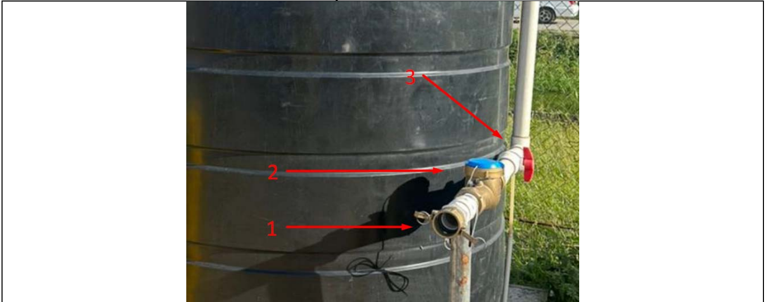
Water supply line setup 1-Cam lock 2- Water flow meter 3- Valve
