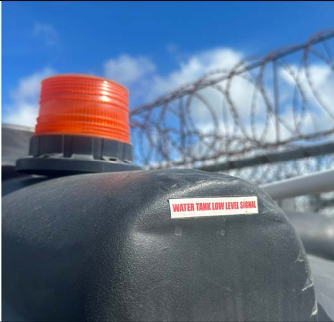
Domestic water tank low level signal
