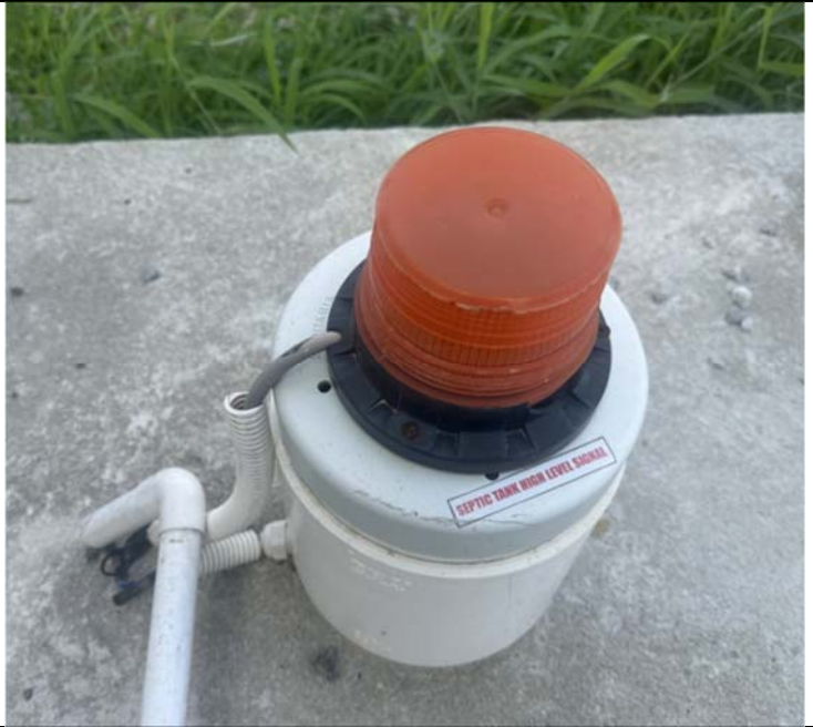
Septic tank high level signal
