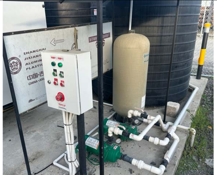
Duplex domestic water pumps with a control panel
