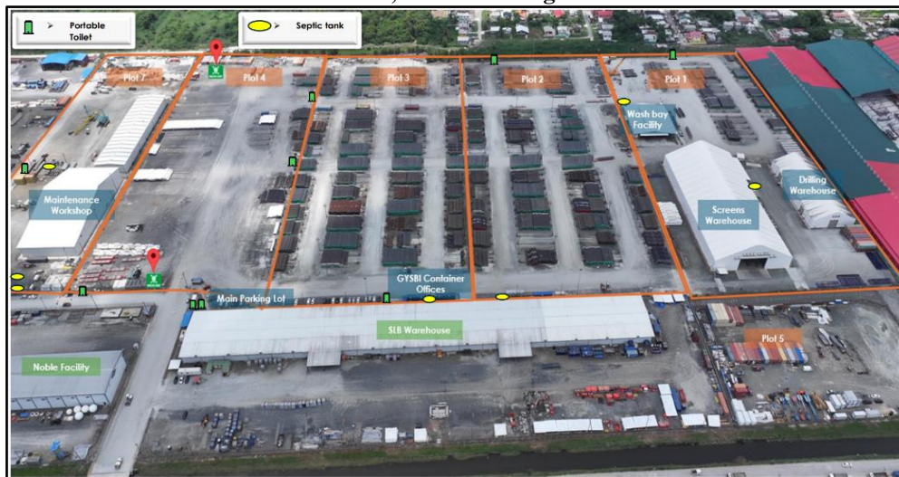
Figure 2: Location of the Sewage Facilities at the GYSBI Industrial Estate Base, Mc Doom, Greater Georgetown.
